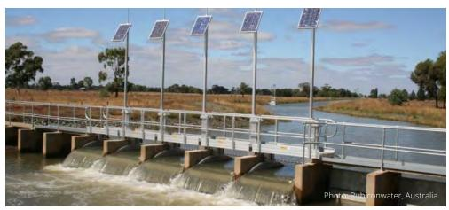
Figure 11 Active automation on a main canal
