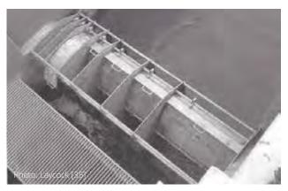
Figure 12 Baffle distributor that delivers a fixed discharge regardless of upstream water level. Variations in flow are made by opening different baffles.
