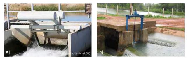
Figure 9 Automatic control of canal water levels a) Floating gate b) Duckbill weir
