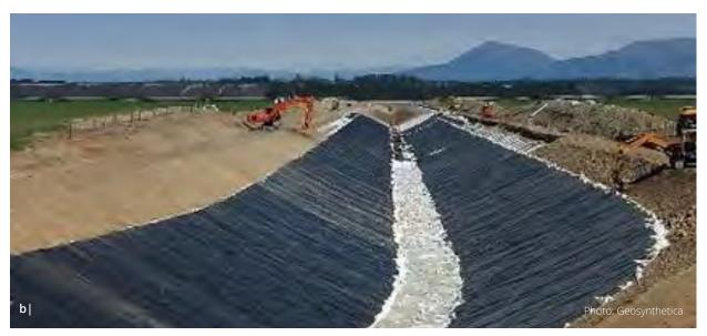
Figure 15 Canal linings a) concrete b) geotextile material
